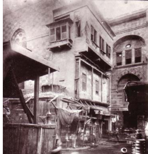
The superstructure before it was torn down by the Comité (courtesy - photographic records of the SCA)
