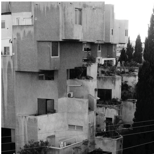
Figure 2: Dubiner Apartment House is a composition of concrete solids, voids and vegetation 16
