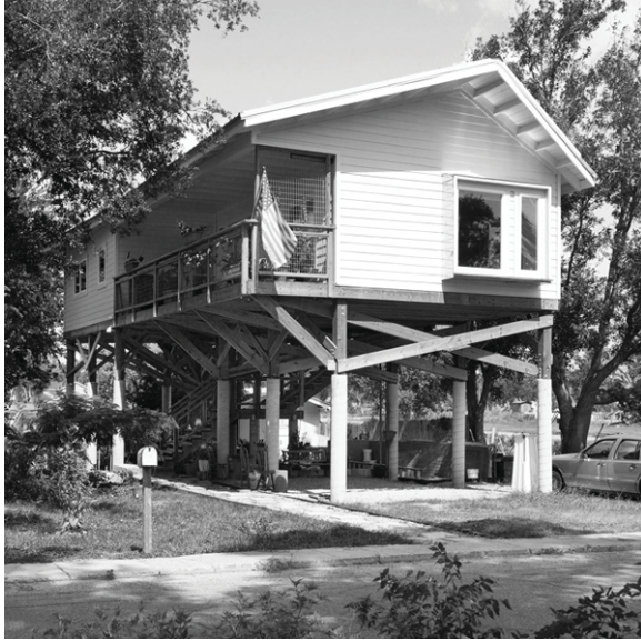
A new GCCDS East Biloxi house elevated 13' above grade. Image © Alan Karchmer 2008
