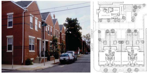
Fig. 4: Project 1800 Phase I: Montgomery and Gratz Streets
