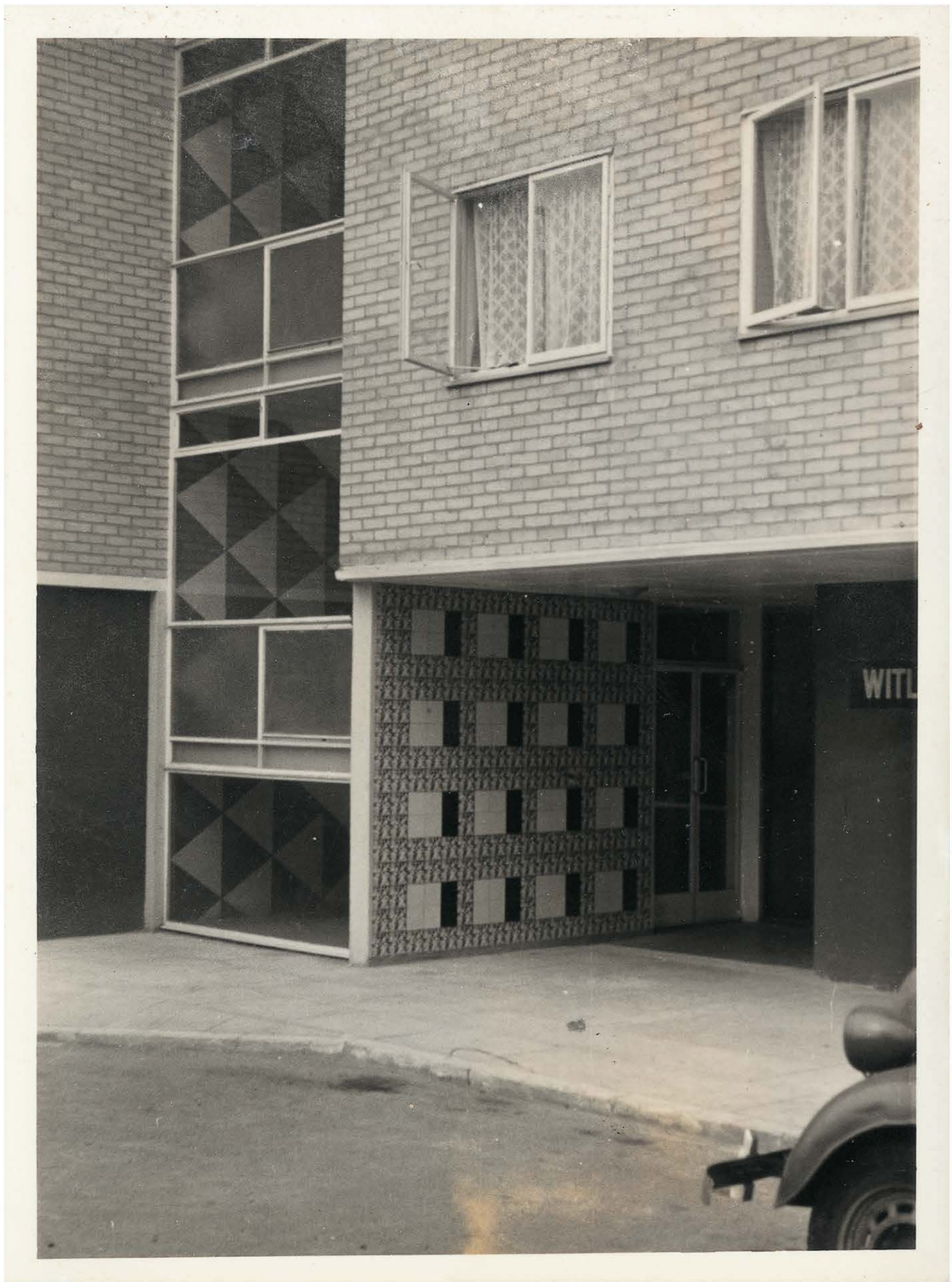
One is particularly damp; the corners are soft, the surface is wrinkled.
