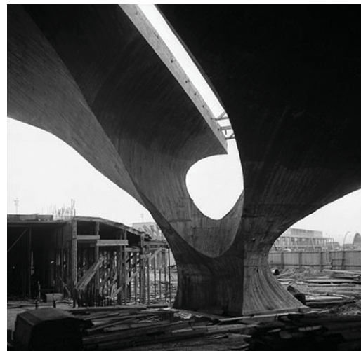
Figure 5: TWA Terminal construction, c. 1960, photograph by Balthazar Korab.
