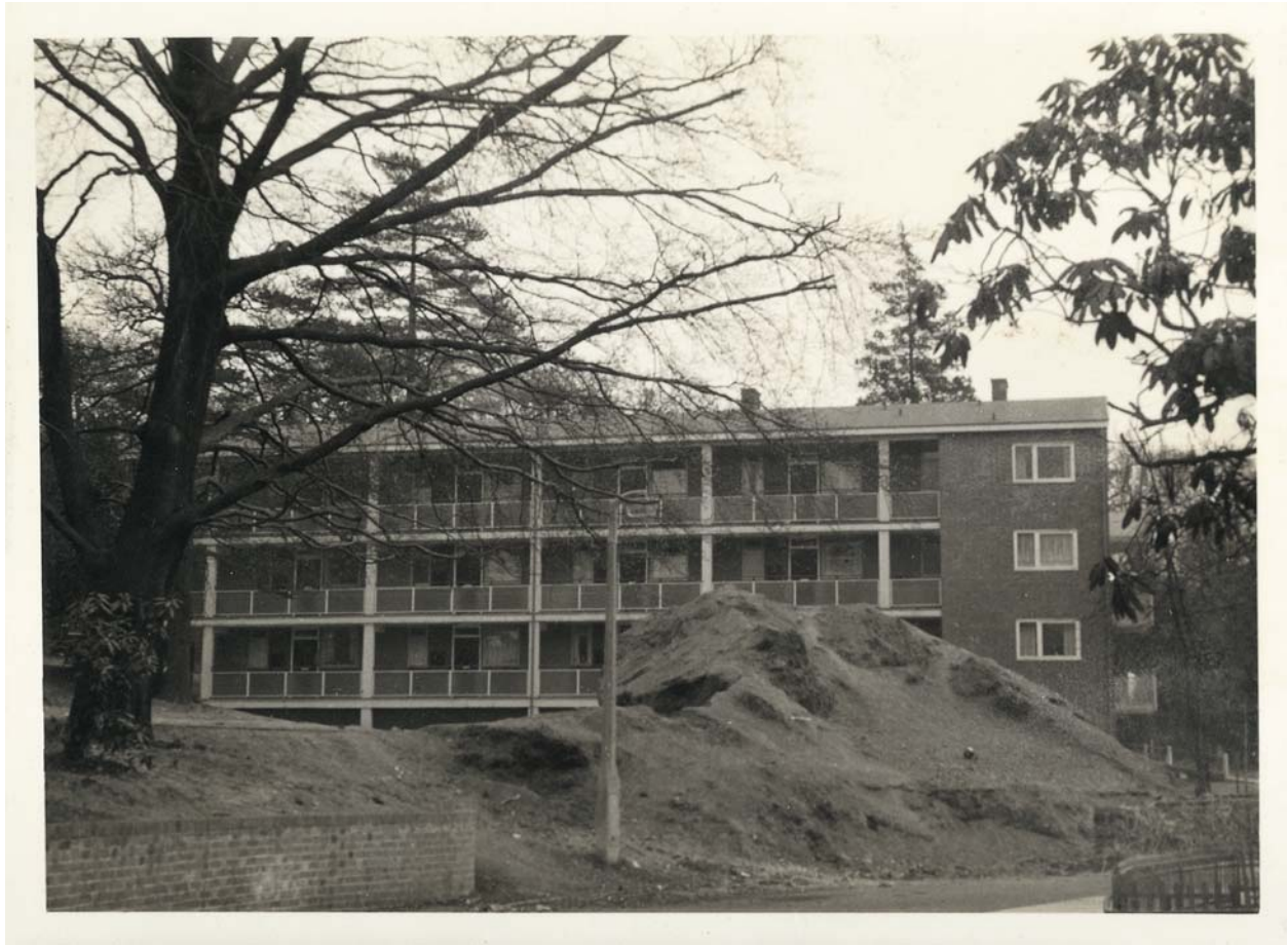
Up close it is clearly derelict, almost in ruins.
